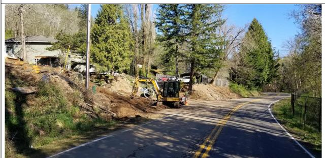
**2.** Another view of the non-permitted development activity being conducted on the property, specifically the extensive non-permitted ground disturbance, grading, site clearing and excavation work, and non-permitted development activity within a stream overlay area.
