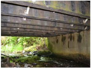
Photos 4 and 5. North elevation showing board-formed concrete wing wall, looking southeast (left). Timber stringers on older concrete abutment (right).
