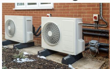
Ans- Yes, we can stop burning fossil fuels for heat by using a Heat Pump, which is a machine that moves heat from a cold place to a hot place.
