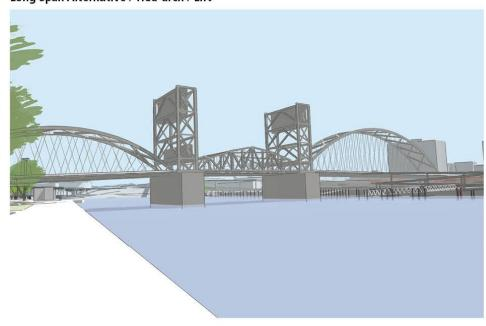
Long-span Alternative / Cable-stayed / Lift
