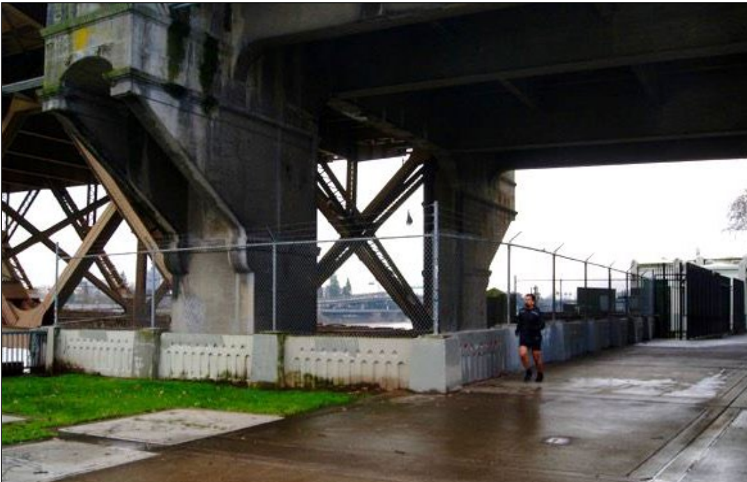
Figure 11. Portland Harbor Wall constructed around Burnside Bridge Pier 1, facing southeast. The original concrete railing panels surround Pier 1 (Elizabeth O'Brien, 2019).
