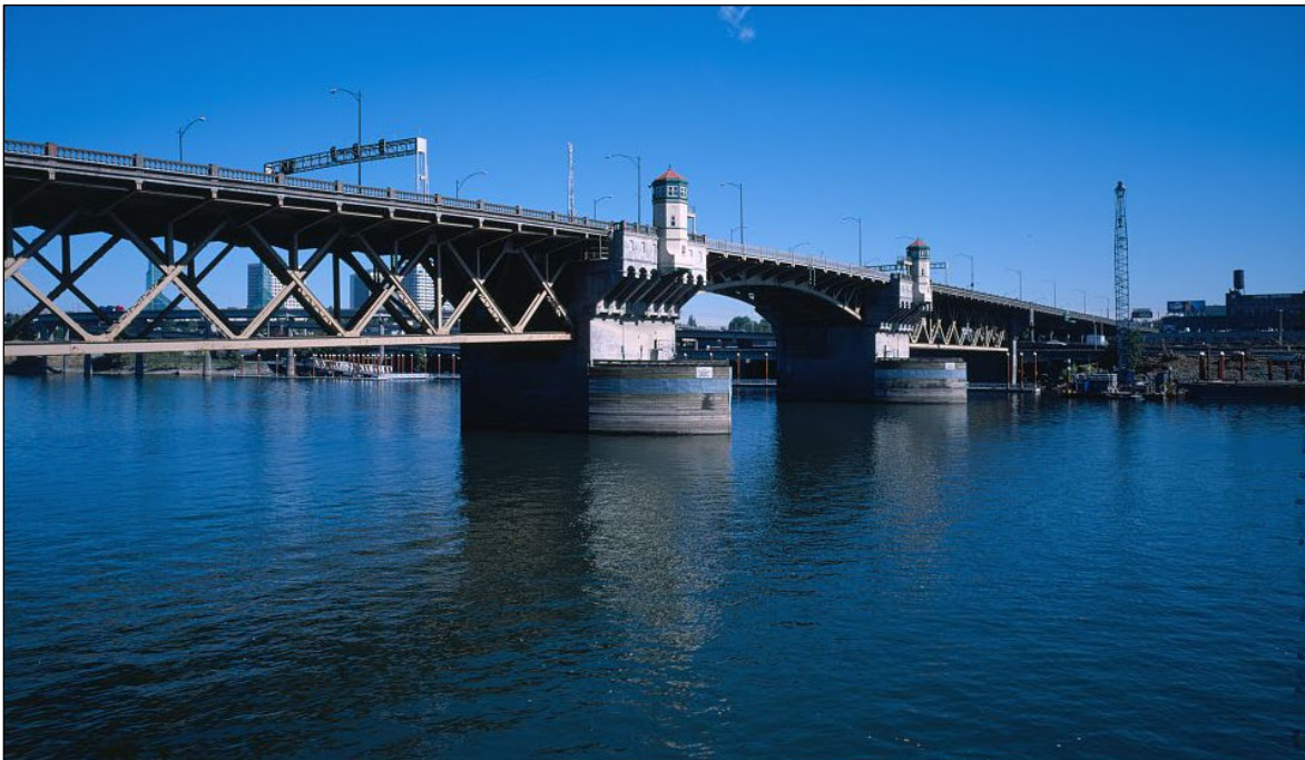
Figure 10: General view of double leaf bascule drawspan of Burnside Bridge, looking northeast. Burnside Bridge, Spanning Willamette River at Burnside Street, Portland, Multnomah County, Oregon. Photos from Survey HAER OR-101 (Library of Congress).
