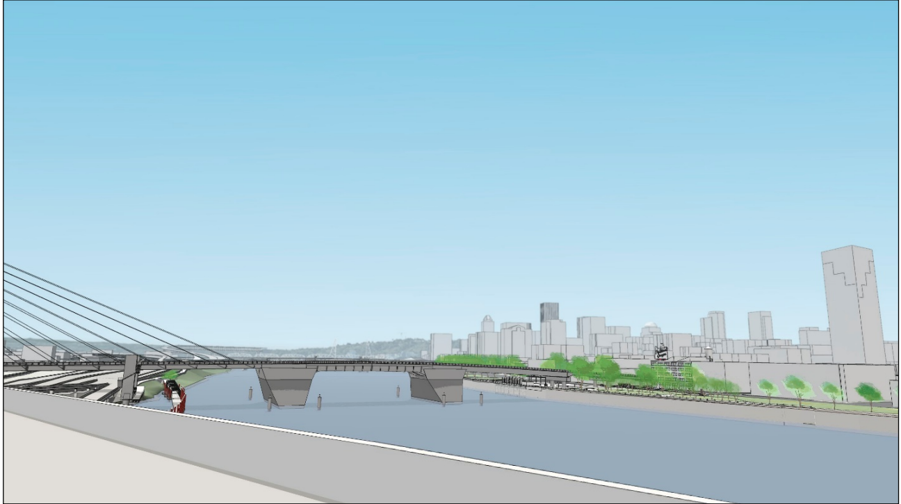
Figure 41: Span Combination 3 (girder west approach, bascule central span, cable supported east approach), artist's rendering, view looking south (Fat Pencil Studio, 2021).
