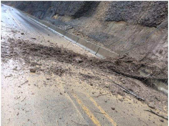
Figure 65 - Minor 2017 winter landslide on the East Historic Columbia River Highway. Photo Multnomah County Sheriff's Office
