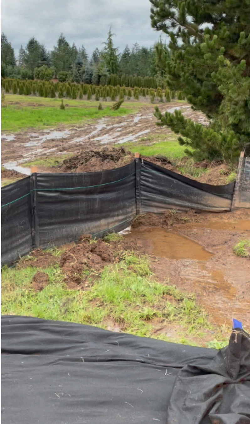
Figure 4. Runoff from a large excavation carried out by PWB's contractors during an assessment on the western edge of the proposed project site looking south. Photo taken two days following a large, five-day storm event totaling approximately 1.5 inches, December 24, 2021. Full video submitted as separate testimony, File name: JCReport-Dec-24-21-Pond.MOV .
