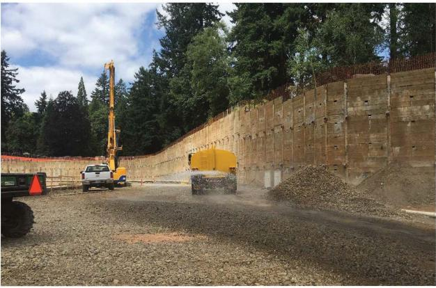
Figure 4. Example of water truck pass to provide dust suppression on gravel construction roads.
