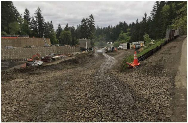
Figure 3. Example of temporary gravel roads and larger construction entrance rock used for onsite construction vehicle traffic. Gravel roads produce less dust than dirt roads.
