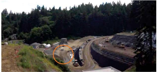
Figure 1. Example of water truck pass to provide dust suppression on gravel construction roads.
