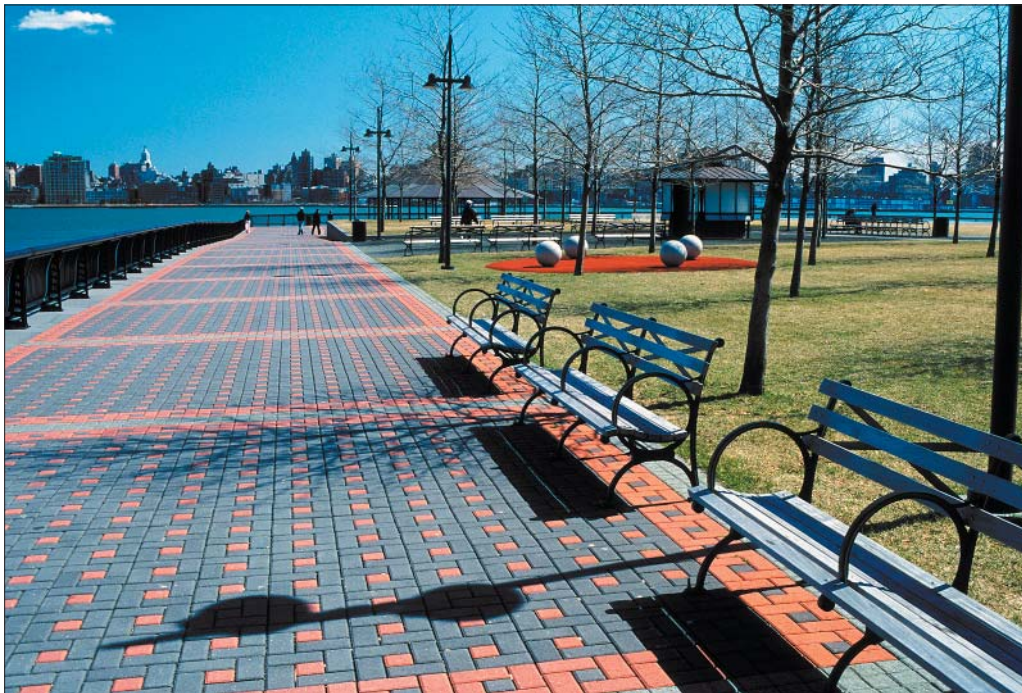
This walkway at the Pier A Park in Hoboken, New Jersey is made with concrete pavers from Capitol Concrete. The 1/4" (6 mm) joints are filled with uniform-size angular aggregate.
