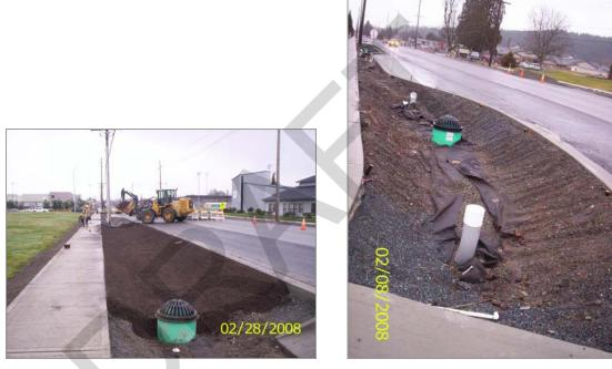
Figure 3. Roadside Green Street /LID Application Under Construction
