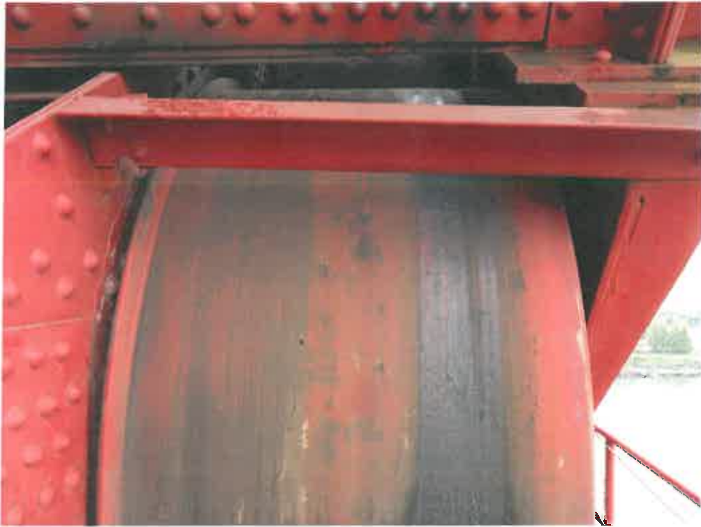
M-045 NE wheel defect (bridge open)
