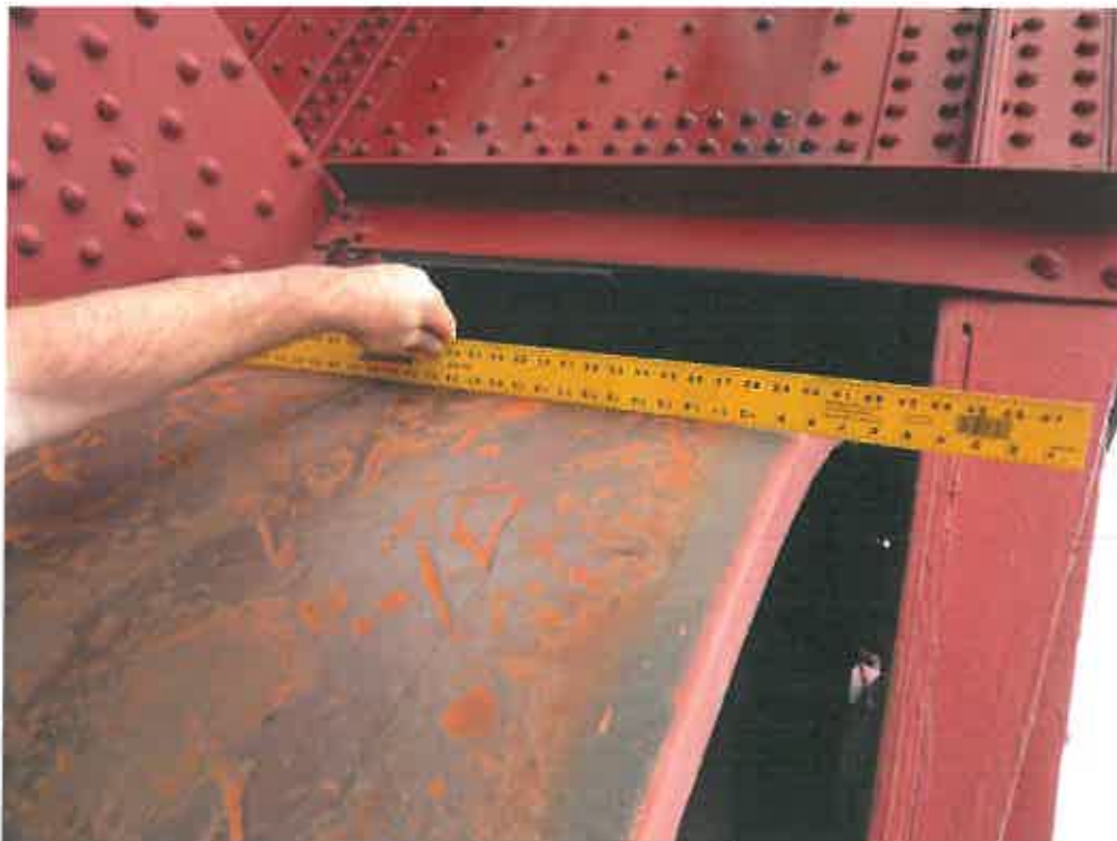
M-040 NE wheel defect
