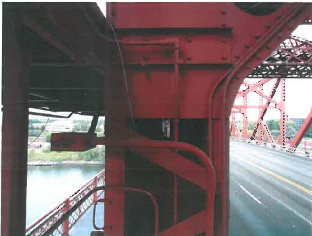
M-064 Column Strain Gage
