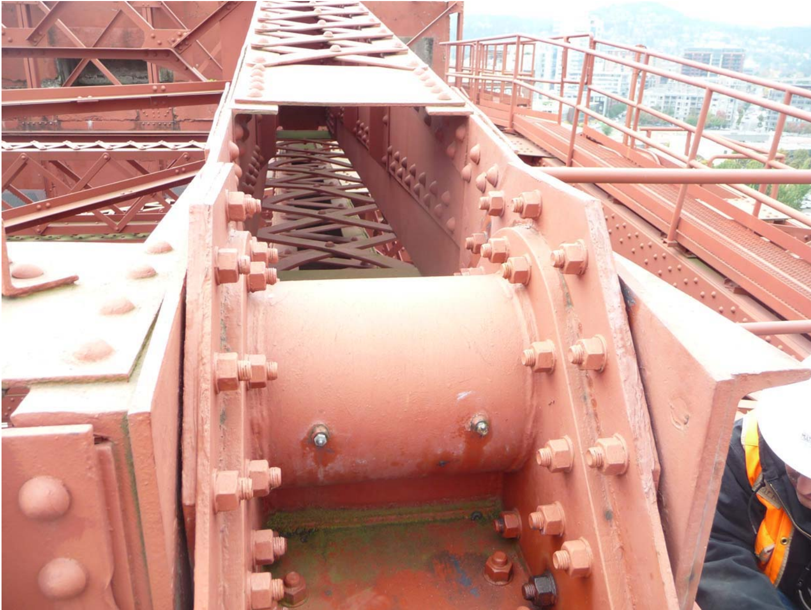
Figure 2 NW OP strut at pinned area 'not' showing rubbing like the SW strut.
