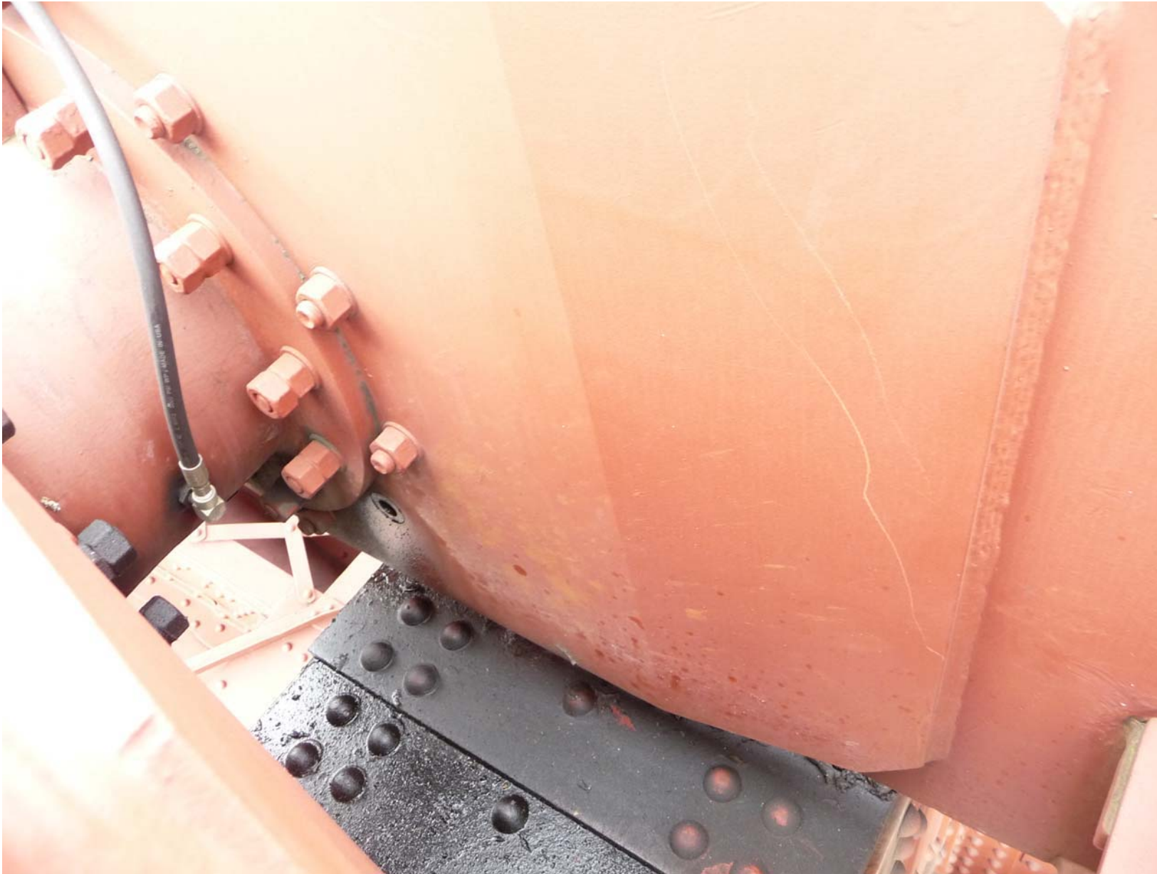
Figure 4 Bolt failure location on Anchor Strut reinforcement plate near Anchor Strut pin.
