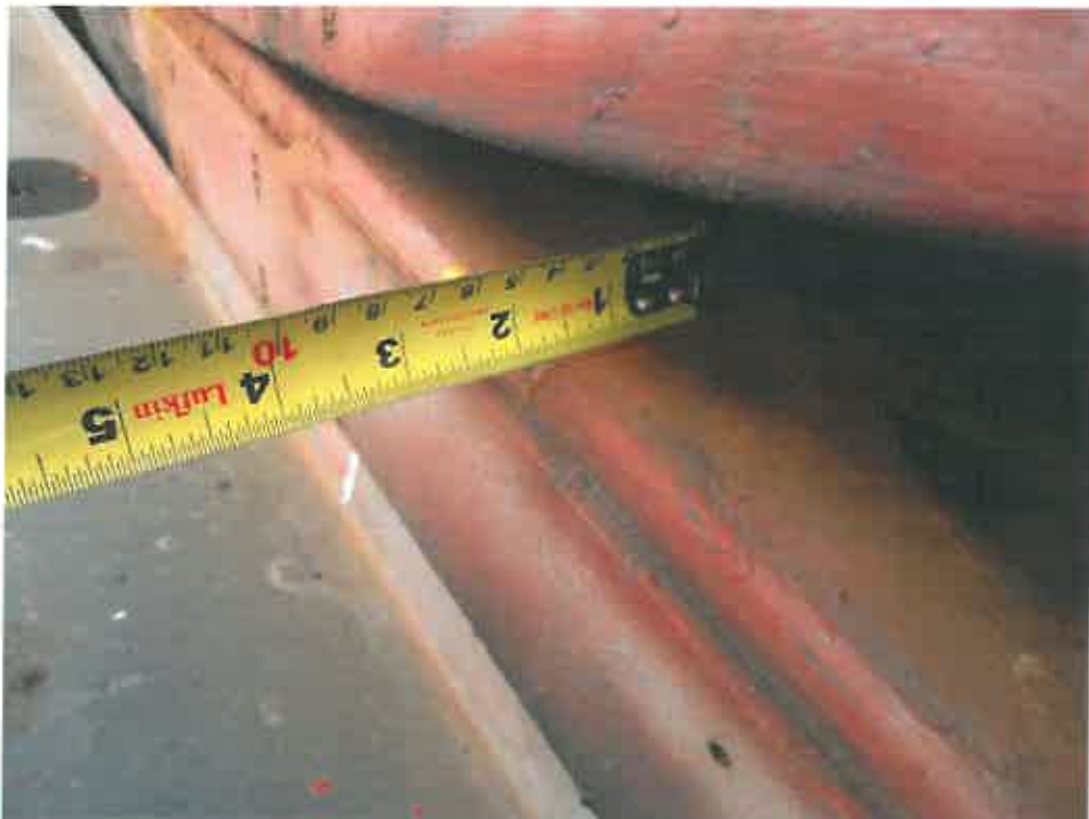
M-060 SE track crack
