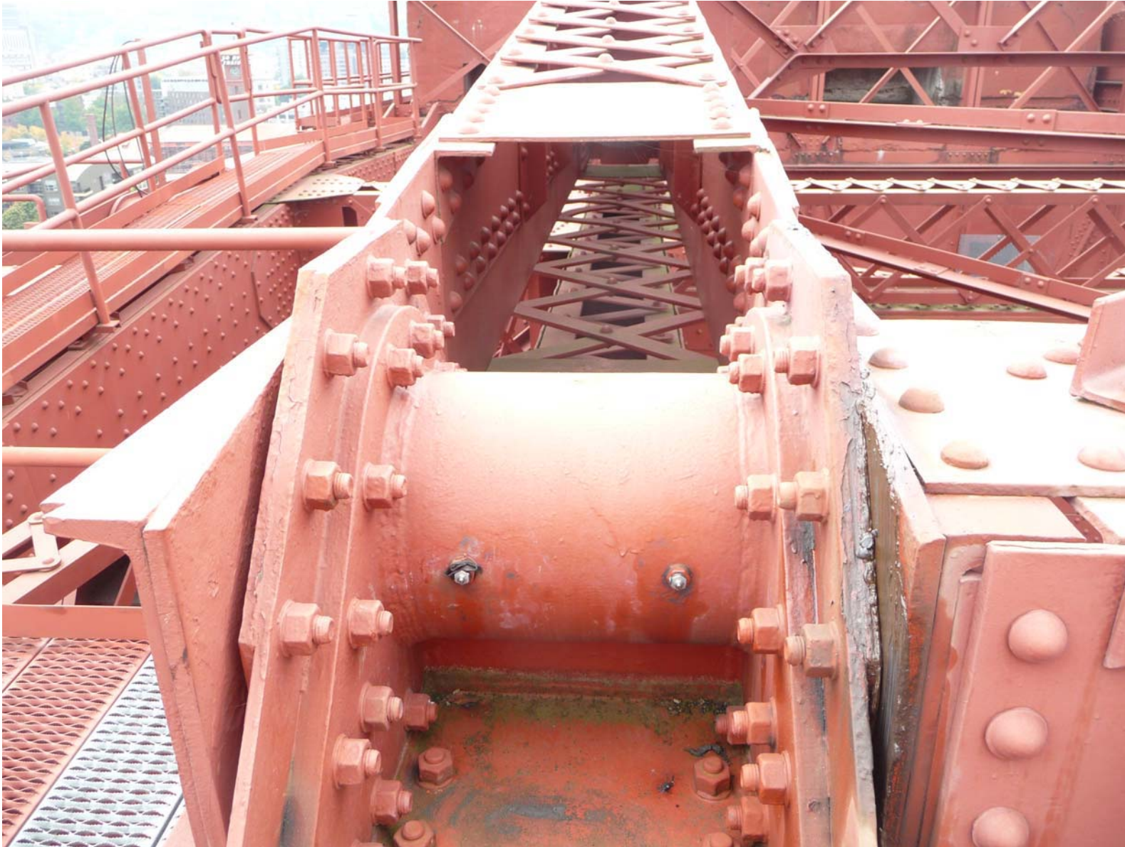
Figure 1 SW OP strut rubbing inboard side at pin. Note grease smeared on metal to metal wearing surface.
