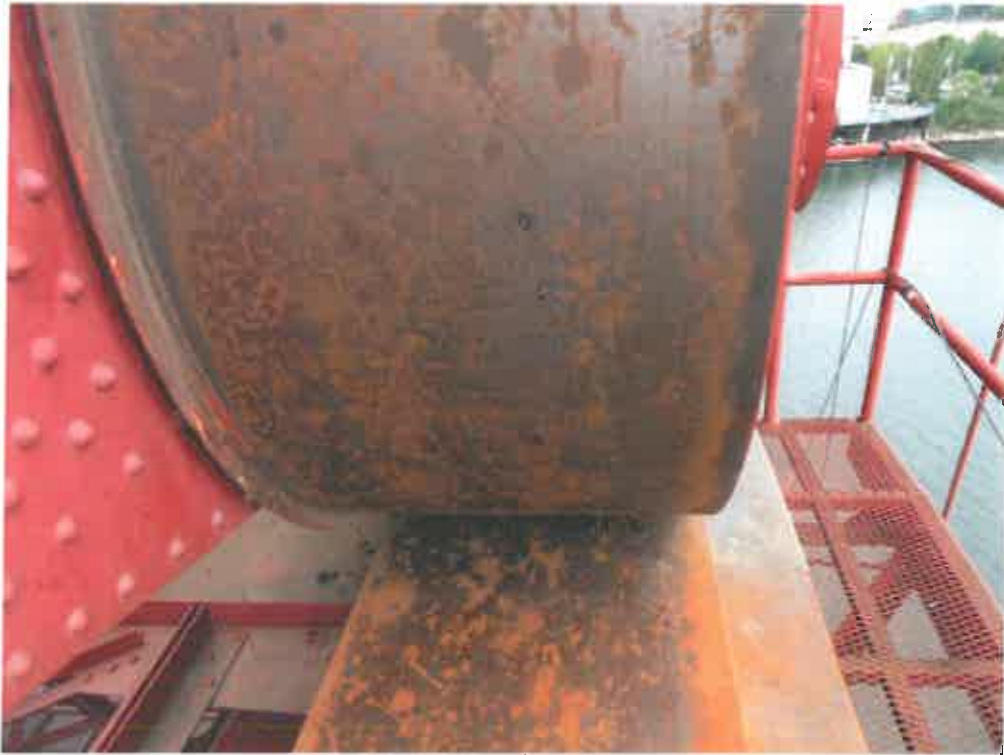
M-039 NE wheel defect
