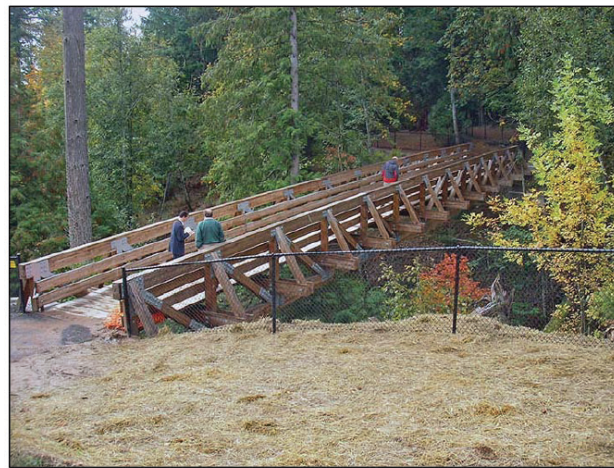
4 EXAMPLE: PONY TRUSS BRIDGE SECTION
