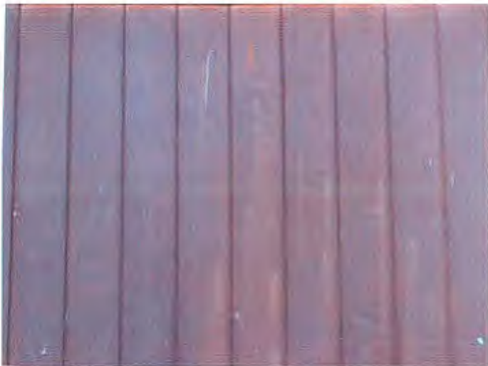
STANDING SEAM COPPER ROOF At New Stair Connection Pre-Patinated for Aged Appearance
