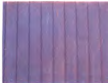
STANDING SEAM COPPER ROOF
