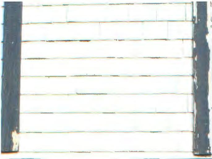
CEDAR SHINGLE SIDING + WOOD TRIM Match existing size - 5 1/4" visible- and texture Match historic black - white color scheme
