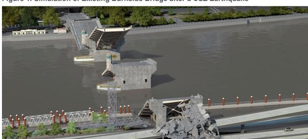
Figure 1. Simulation of Existing Burnside Bridge after a CSZ Earthquake
